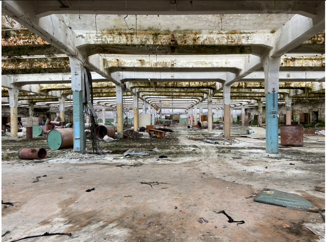
Spinning mill from approx. 1890, northern interior, looking north. Photo: Ivo Hammer 2021
