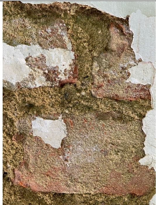
Schindler's Ark, 2nd floor, reinforced concrete hall, northern annex room, view to the south, detail: bricks, brownish masonry mortar, yellowish white lime whitewashes. 1-2 later whitewashes. Photo: Ivo Hammer 2021
