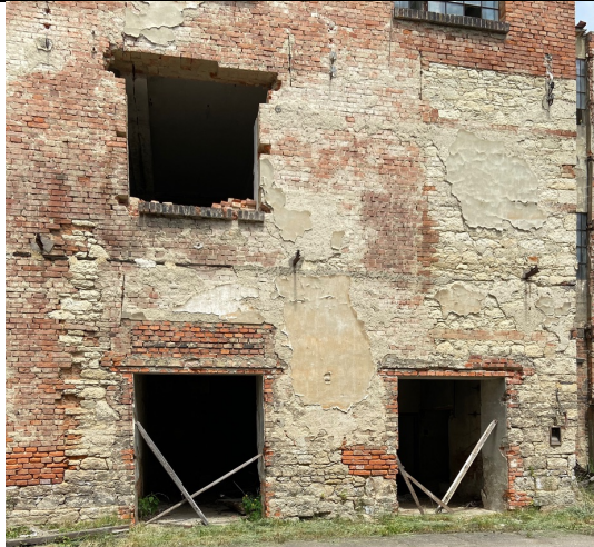
Brnec, Schindler's Ark, south facade, east corner, lower part.
