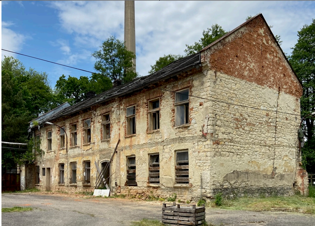
Former laboratory and workshop (SS-Bau des KZ Brnenec, German building). 2 construction phases: stone masonry mixed with bricks, 2 storeys. Gable wall built with brick. The windows on the upper floor possibly enlarged with brick, with a wedge-shaped brick lintel. Both gable walls raised. 2 chimneys in the east. Roof covered (2012?), Only the roof battens left. Completely devastated inside. Remains of plaster and whitewash preserved on the south facade. Window frames and window sashes still partially preserved. Photos: Ivo Hammer 2021
