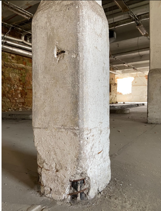
Schindler's Ark, 2nd floor, reinforced concrete hall, view to the southeast, detail: reinforcement of the pillar with reinforced concrete. Photos: Ivo Hammer 2021
