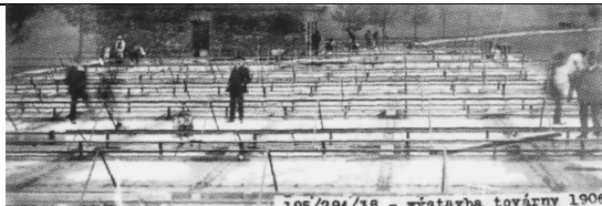
Construction of a weaving hall (Moses Löw-Beer company) in Ingrowitz (Jimramov-Benátky), 1906. Photo from PS 2017, p. 125 (Pavel Novotný archive)
