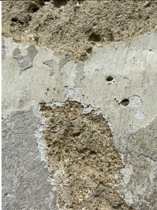
Former laboratory and workshop (SS-Bau des KZ Brnec, German building). Details of the south facade (lower edge of the picture approx. 10 cm). Base plaster with yellowish-gray mortar with fine lime sparrows (dry slaking),
