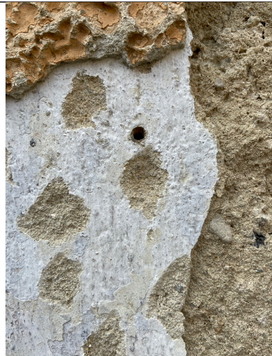
Rubbed surface, very light yellowish-white, thin Freko whitewash. 2 thin yellowish-white whitewashes. Stubby plaster with light gray mortar with fine lime sparrows, possibly natural plaster 3 whitewashes: brown, light red-brown, green. Photos: Ivo Hammer 2021
