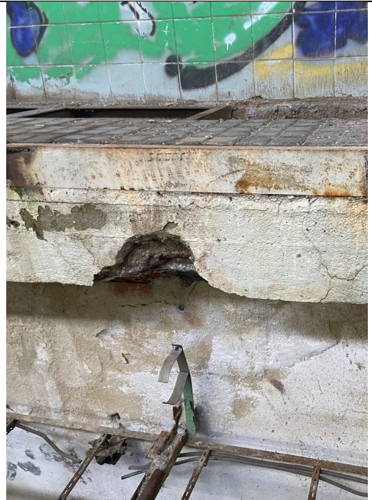
Schindler's Ark, dye works, concrete reinforcement
