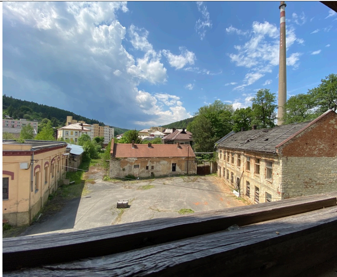
Brněnec, view from the upper floor of the former spinning mill II (Schindler's Ark) onto the courtyard (Brněnec concentration camp) with former carding (left), former residential building (administration Oskar and Emilie Schindler), former laboratory and mechanic's workshop (SS building). Photo: Ivo Hammer 2021
