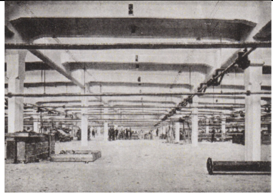
Southern area (?), Newly built hall according to the Hennebique system, around 1900. Photo: after r21 architects
