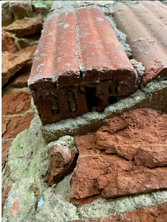
Detail of the walling up of the window
