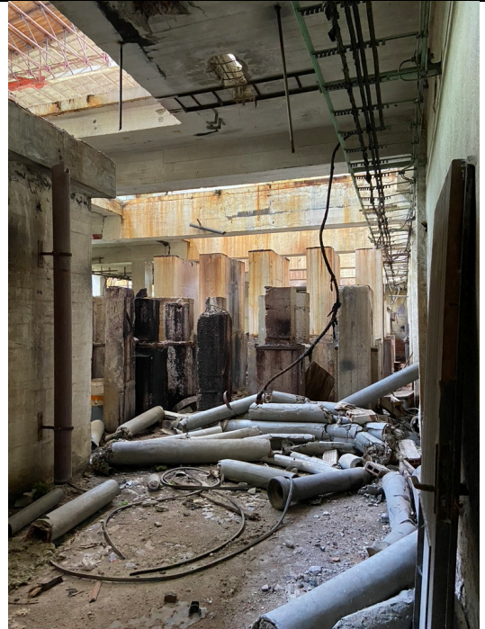
Dyeing works, ground floor, with bases of the dyeing centrifuges. Photos Ivo Hammer 2021
