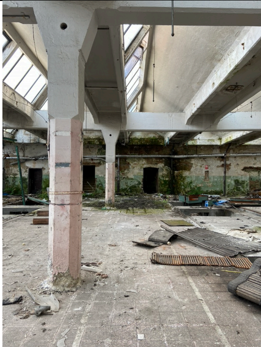
Spinning mill from approx. 1890, north interior, view to the east. Photo: Ivo Hammer 2021
