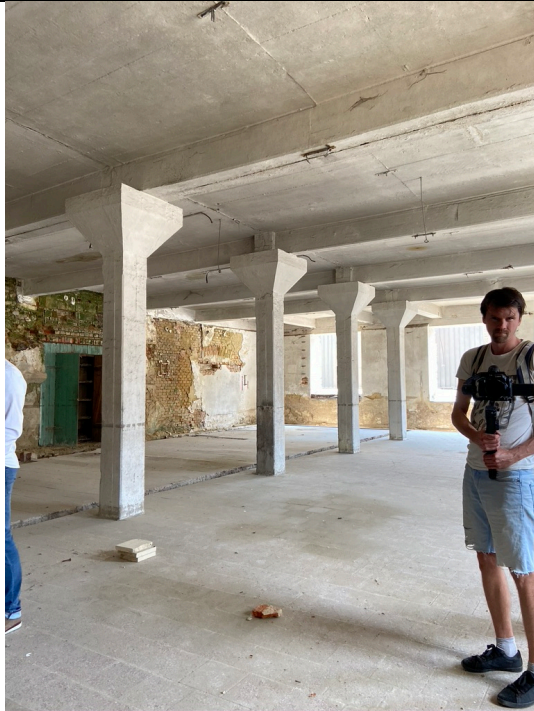
Schindler's Ark, ground floor, reinforced concrete hall, built into an older structure. View to the southeast. Photos: Ivo Hammer 2021
