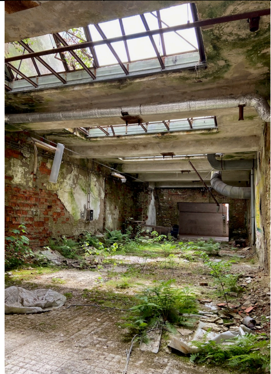
Schindler's Ark, 2nd floor, space between the reinforced concrete hall and the dye works, view to the southeast, reinforced concrete ceiling with hypäthral light.
