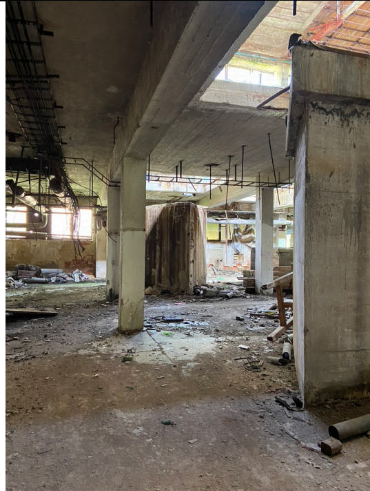
Dyeing works, ground floor, with bases of the dyeing centrifuges. Photos Ivo Hammer 2021
