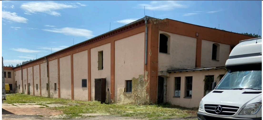
Spinning mill, north and east facade. Photo: Ivo Hammer 2021
