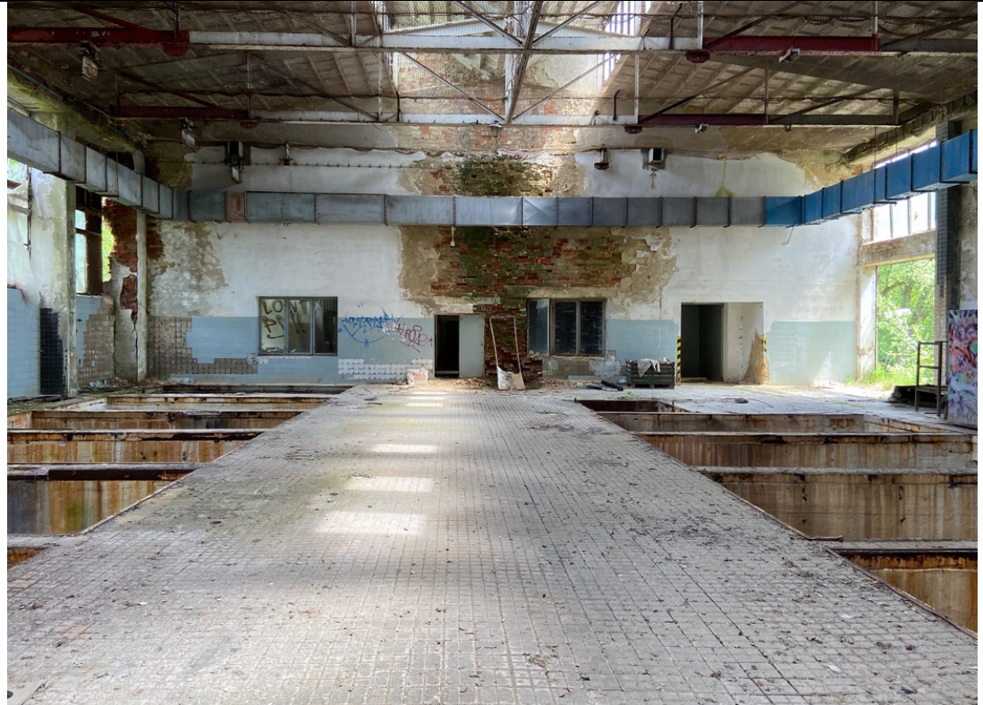
Schindler's Ark, dye works, looking east. Concrete tiles of the floor with wedge joints. The steel structure of the roof with ribbon windows opening to the north and south. Photos: Ivo Hammer 2021
