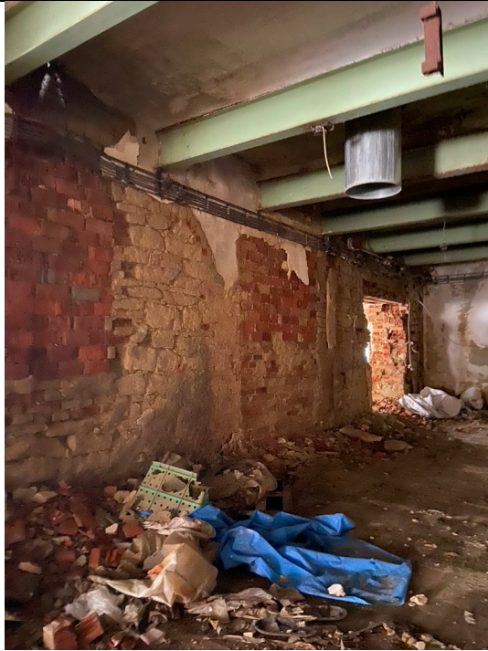
Schindler's Ark, ground floor, room east of the reinforced concrete hall. Stone masonry rebuilt with bricks.
