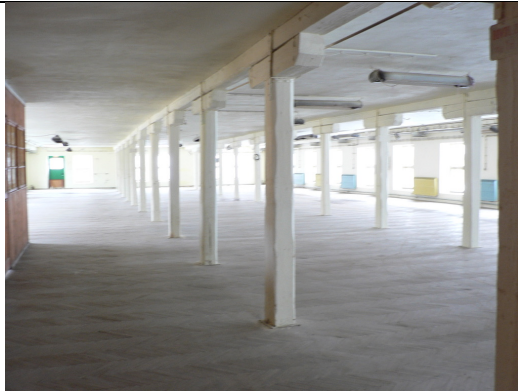
Old hall with wooden architecture, after 1854. Photo: Archives Frantisek Olbert, approx. 2010
