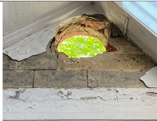
Spinning mill from approx. 1890, southern interior, western oculus of the gable wall of the hypäthral light. The inside of the gable wall is coated with panels that are black at the break edge. Possibly slag and bitumen or cement (?) Panels. The panels are probably used for thermal insulation. Photo: Ivo Hammer 2021
