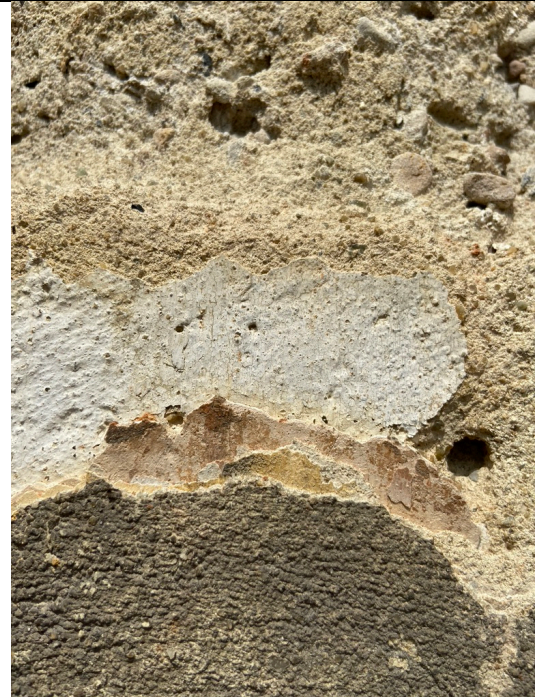
Fine plaster with the same mortar, only finer grain. Rubbed surface, very light yellowish-white, thin Freko whitewash. Approx. 5 whitewashes. Recent rub from (lime) mortar. Photos: Ivo Hammer 2021
