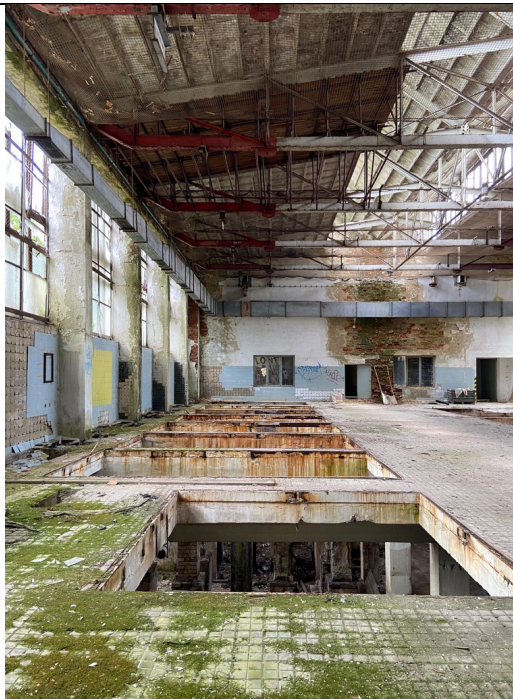
Schindler's Ark, dye works. Reinforced concrete construction with large north windows, facing south, closed towards the annex. Reinforced concrete floor with openings for the centrifuges,
