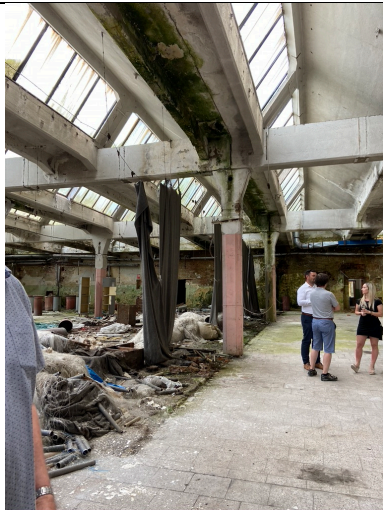
Spinning mill from approx. 1890, northern interior, joint between two yoke compartments in the side member and the cross member. In this area, the pillar is not monolithically connected to the girders. Photo: Ivo Hammer 2021
