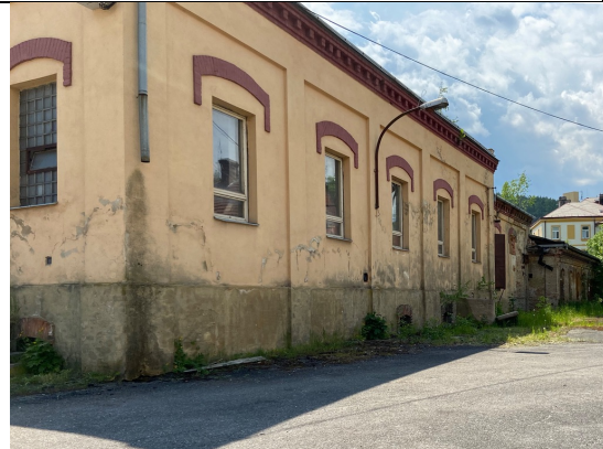
Carding?), View from the northeast. Around 1900? With pilaster strips, segment-arched crowning of the windows, profiled brick eaves with tooth cut, smooth (cement?) Plaster, whitewashed yellow. Flat roof. Crowning the east facade. Photos: Ivo Hammer 2021
