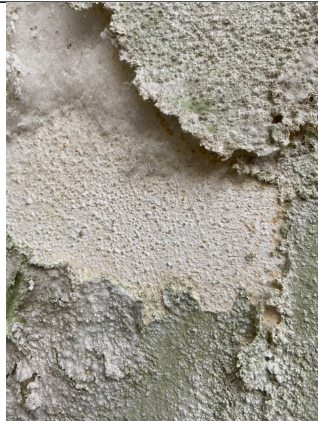
Spinning mill from approx. 1890, northern interior, detail of the west wall. Possibly original rubbed and whitewashed surface. Photo: Ivo Hammer 2021
