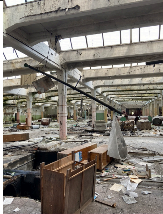
Spinning mill from approx. 1890, northern interior, machine pit and the rest of the heating pipes below the cross member. Photo: Ivo Hammer 2021
