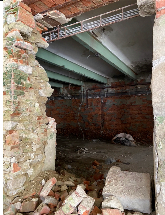
Schindler's Ark. View of the adjoining room to the east: ceiling made of double T-beams with vaulted spaces.
