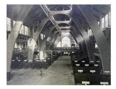
Breslau Market Hall (Hala Targowa) 1906-1908, Architects: Richard Plüddemann and Heinrich Küster Reinforced concrete, the facade clad with exposed bricks, plaster and natural stones, "simple painterly treatment of the interior surfaces of the hall whereby the concrete color of the supporting structures is retained and an element that is foreign to the building material is not brought into it by plaster and plastering work."10 Photo: Ivo Hammer, 2009, after a historic photograph on site
