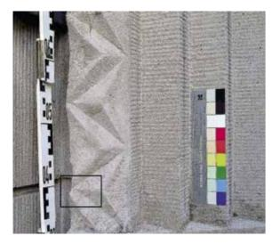
Peine, Lessing Lodge, west facade, entrance area / stucco edging. Condition after the repair. The repair plaster adapted very well in color and structure to the original material. Photo: HAWK / Götz, 2007.
