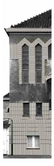
Peine, Lessing Lodge, east facade, base, detailed view: cast concrete plaster with horizontal joins and dressed treatment by chisel. Photo: HAWK / Götz 2007.
