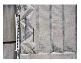
Peine, Lessing Lodge, west facade, entrance area / stucco edging. Damage in the cast stone. The corrosion products on the iron reinforcement were removed with the sandblaster. Photo: HAWK / Götz. 2007
