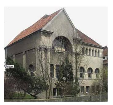
Peine, Lessing Lodge, east facade. Representative design of the facade by changing the surface arrangement; (blue): scratched plaster: vellow: cast concrete plaster, dressed by a stone mason using a charring chisel; (green): dressed concrete, partly prefabricated before transferring it to site. Photo / graphic: HAWK / Götz. 2007.
