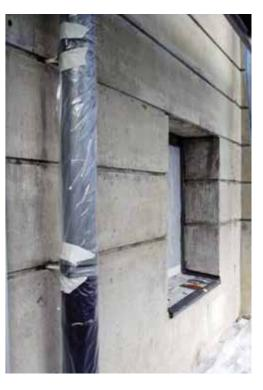
and incrustations could not be removed even in a second cleaning cycle. In order to be able to clean these areas, the cleaning paste was modified. A 20% pure ammonium carbonate solution replaced deer horn salt, mixed with 4% Tylose® and 50 g beech cellulose Arbocel BC 200®.36
