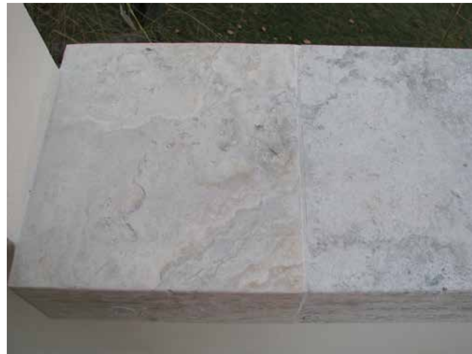
Brno, Tugendhat House travertine covering the parapet of the upper terrace; left: after chemical cleaning, right: cleaned with steam jet only. Photo: Ivo Hammer 2011
