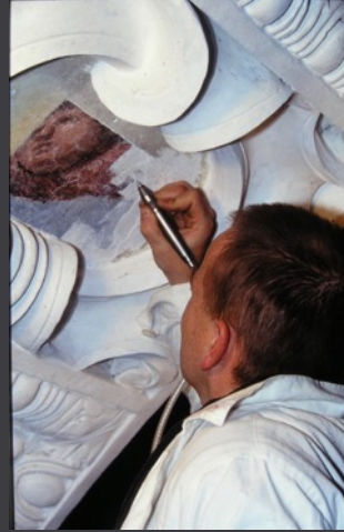
Mariabrunn, triumphla arch, uncovering of ceiling paintings, scalpel, Pneumatic microcise 1990
