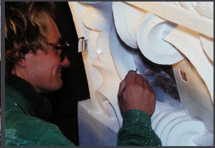
Mariabrunn, triumphla arch, uncovering of ceiling paintings, scalpel, Pneumatic microcise 1990
